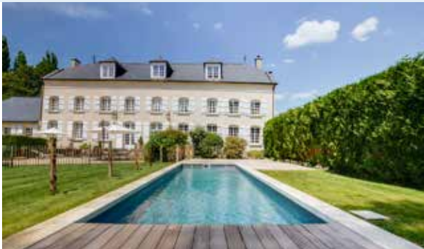
10x3.5 in Saint-Etienne Roilaye, pool installation by Piscine Emois.
