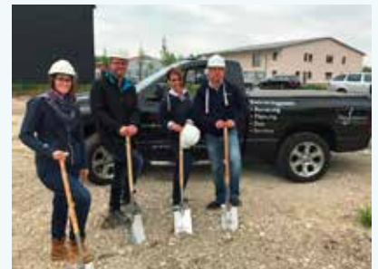
Launch of building work on the new subsidiary headquarters in Neufahrn, Germany.
